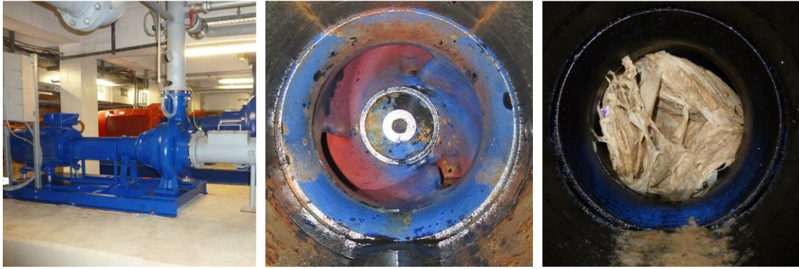
Figure 3-3: From left to right: Wastewater pump from which blockages were collected; view into the impeller of the pump; view into the clogged impeller
