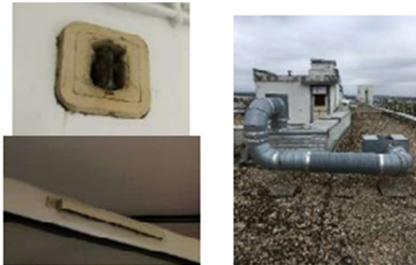
Figure 10: Ventilation and the galvanized ducts
