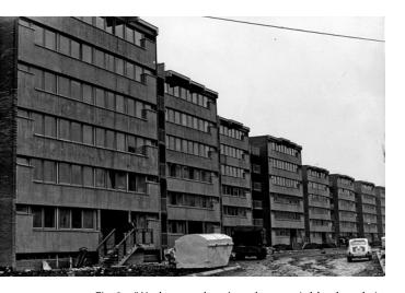
Fig. 3: 'Workers colony'—urban neighborhood in Kruševac, Serbia, built around 1975 in a modified version of *Jugomont YU-61* panel system. Because of the aluminum parapets, the buildings are called 'tins'.
