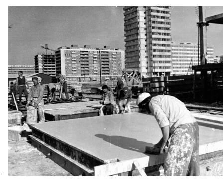
Fig. 1: Construction site, Blocks 1 and 2 in New Belgrade: workers are casting the slab manually (IMS system—GP Naš Rad)
