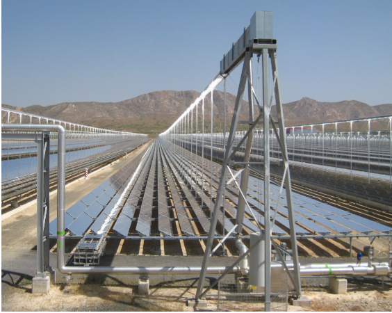
Figure 2.3: Novatec LFC collector, Puerto Erado, Spain
