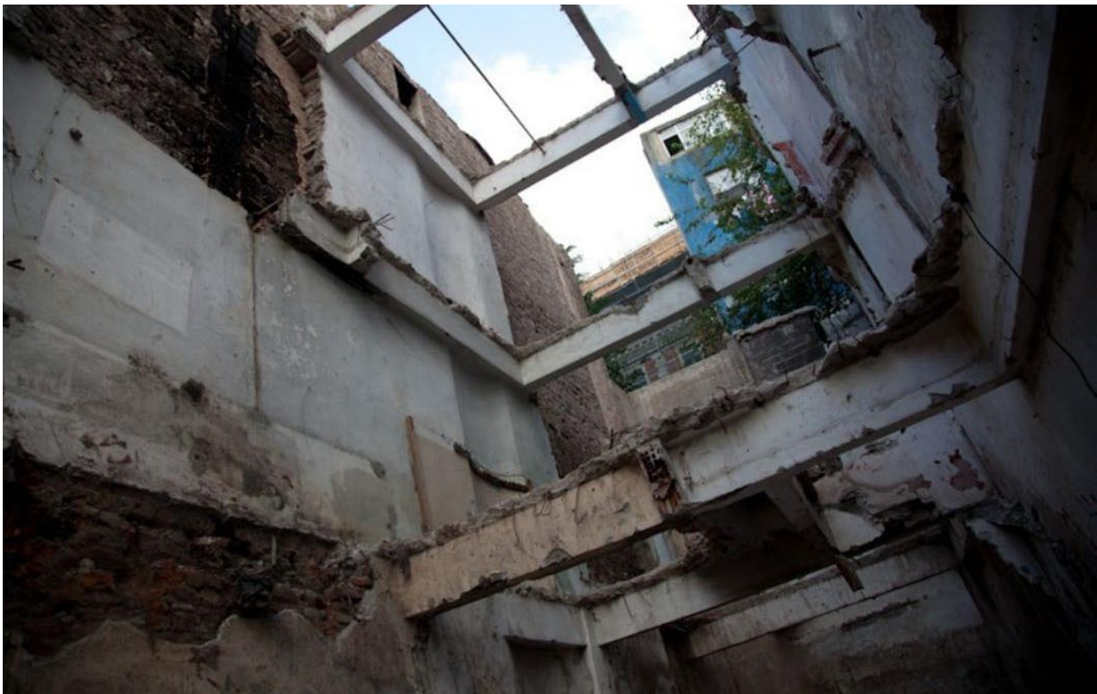
Figure 33: Demolished House with remaining Minimum Supporting Structure, Source: Jonathan Lewis, 2011
