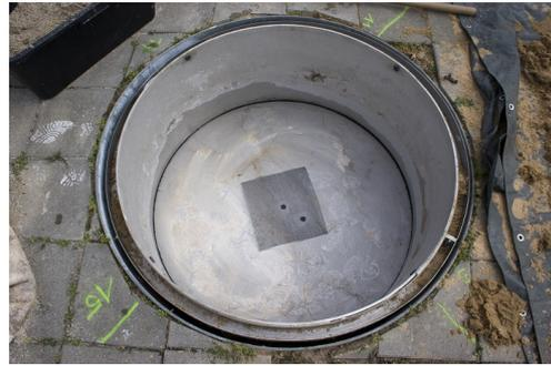
(b) mesh protecting infiltration outlet
