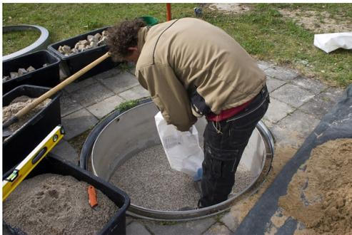
(c) installation of gradient drainage layer
