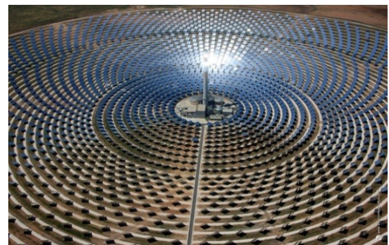
Figure [3-5]: Gemasolar 20MW CSP plant Source: (Andrews, 2016)
