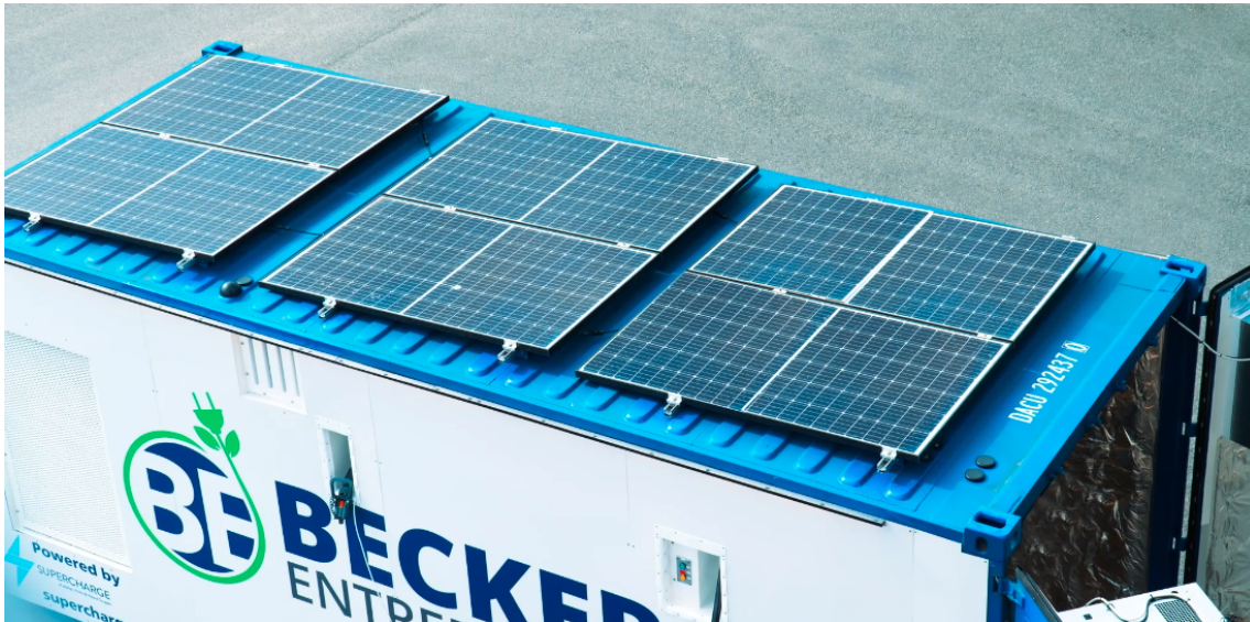
Figure 2.2: Solar panels on construction site BESS
