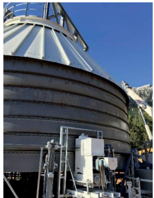
Figure 10. Welded tank with stiffeners: cross section of the tank wall (a), welded tank in construction stage (b) (Lipp company, Tannhausen, Germany).
