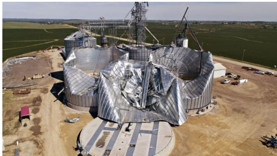
Figure 2. Damaged silos after a storm, Marshalltown, Iowa, USA, 2020 [2].
