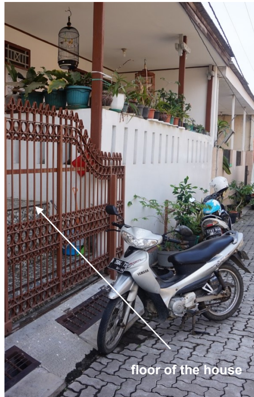
Picture 2: House in Kel. Panggung Lor whose floor had been lifted for 3m in total. (Picture: Ziegelmayer 2015)
