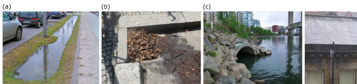
Figure 2.6: Buffers, barriers, and boosters of urban diffuse pollution: (a) swale directly after rain event, (b) blocked gully, and (c) stormwater outlet and rain gutter.
