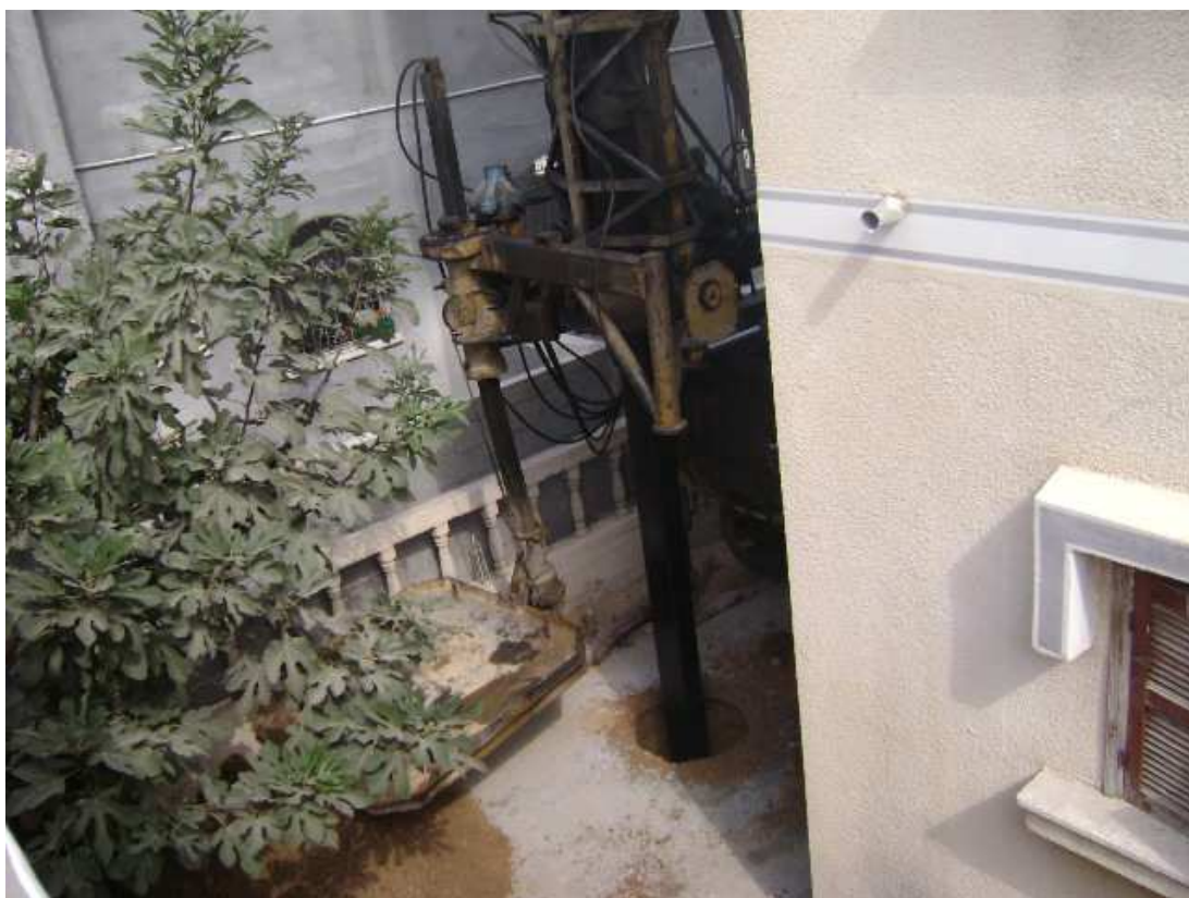
Fig. 3.4 Drilling for infiltration pit close to pilot house
