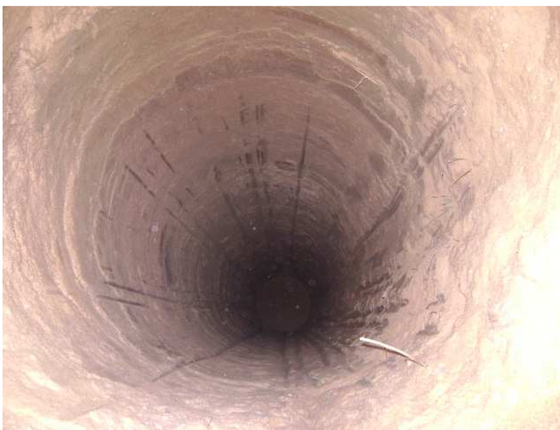
Fig. 3.5 Drilled borehole (8 m) depth until Kurkar (sandstone) layer reached
