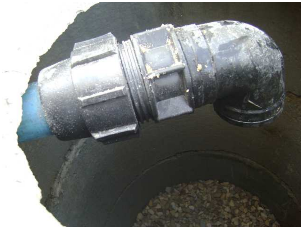
Fig. 3.9 Infiltration pit for rooftop rainwater
