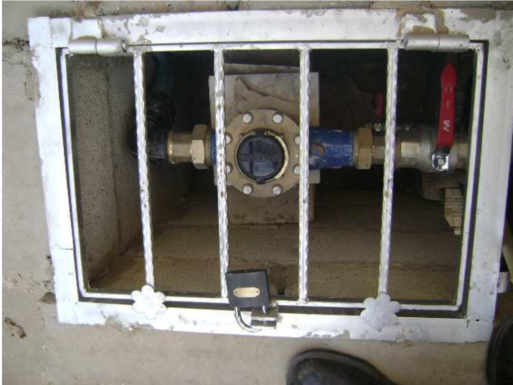
Fig. 3.8 Flowmeter between storage tank and first infiltration pit
