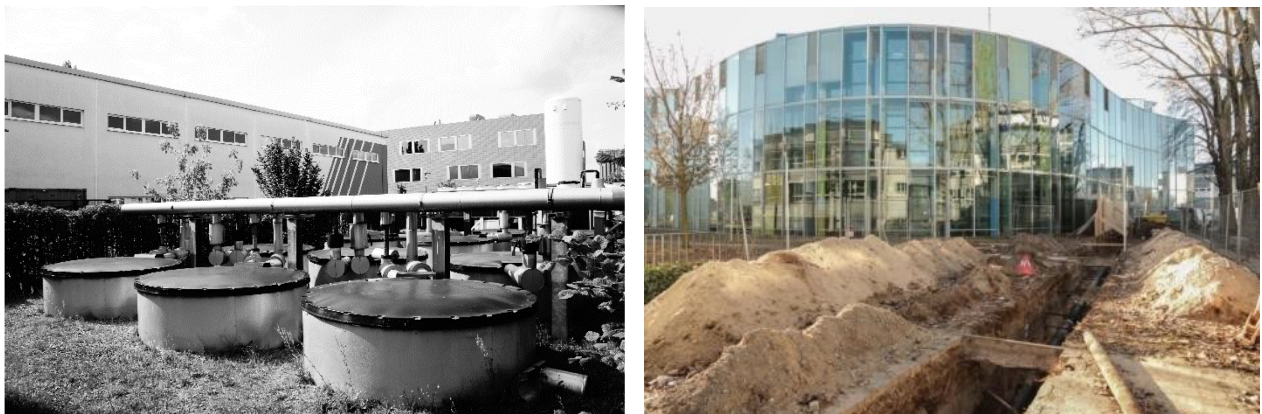
Figure 17: Ice storage facility at ZPO © TU Berlin (left) and cooling network being connected to ZPO © Energienetz Adlershof (right)
