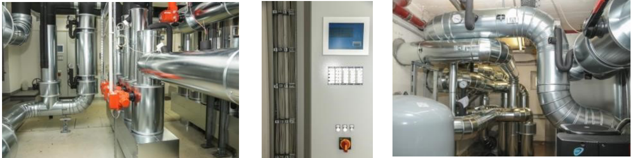
Figure 18: Newly constructed cooling distribution system with information point © TU Berlin
