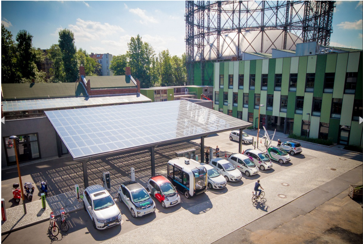
Figure 21: Photovoltaic roof and electric vehicle charging stations at EUREF Campus © InnoZ / Vipul Toprani
