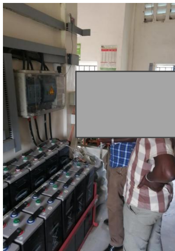
Picture A8: Inspection of the batteries, charging system and inverters at the Mbita Hub
