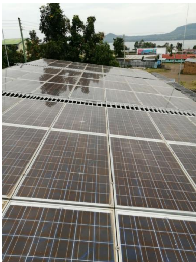
Picture A7: Solar panels on the roof of the Mbita hub
