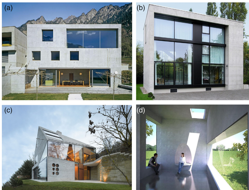
FIGURE 2 (a) Lightweight concrete (Gartmann house) Schweiz 2003 density; 1,100 \text{ kg/m}^3 , thermal conductivity; 0.32 \text{ W m}^{-1} \text{ K}^{-1} , strength; 12.9 \text{ MPa} [13]. (b) Infra lightweight concrete (Schlaich house) Berlin 2007 density; 760 \text{ kg/m}^3 , thermal conductivity; 0.18 \text{ W m}^{-1} \text{ K}^{-1} , strength; 7.4 \text{ MPa} [32]. (c) Lightweight concrete (house H36) Stuttgart 2012 density; 1,000 \text{ kg/m}^3 , thermal conductivity; 0.23 \text{ W m}^{-1} \text{ K}^{-1} , strength; 10.9 \text{ MPa} [13]. (d) Infra lightweight concrete (Pavilion) TU Eindhoven 2015 density; 780 \text{ kg/m}^3 , thermal conductivity; 0.13 \text{ W m}^{-1} \text{ K}^{-1} , strength; 10 \text{ MPa} [13]
