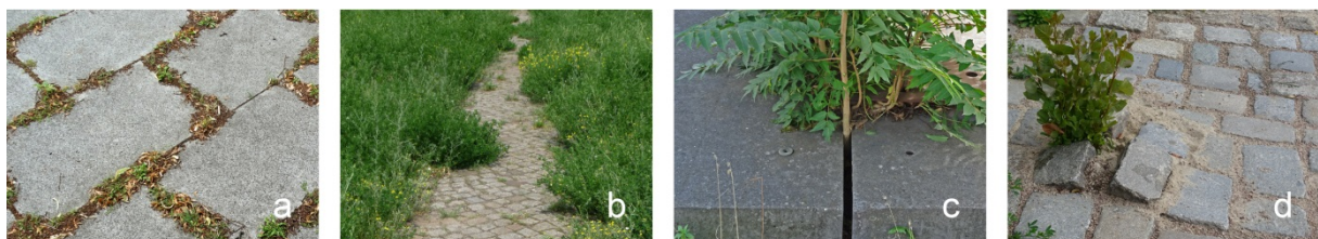
Figure 1: Consequences of spontaneous urban growth on the built landscape. a) Filling of joints, cracks, fissures and recesses, b) Encroachment and spreading of plantings over surfaces and boundaries resulting in the veiling of structures, c) Leverage effects through root wedging and heave leading to further weathering, d) Loss of functionality, usability, stability or safety.
