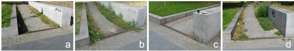
Figure 5: Spontaneous growth between short walls over 8 years. a) Spontaneous growth at the base of short walls, Years 3. b) Year 6. c) Removal of growth in year 7. d) Rapid regrowth of vegetation in year 8.
