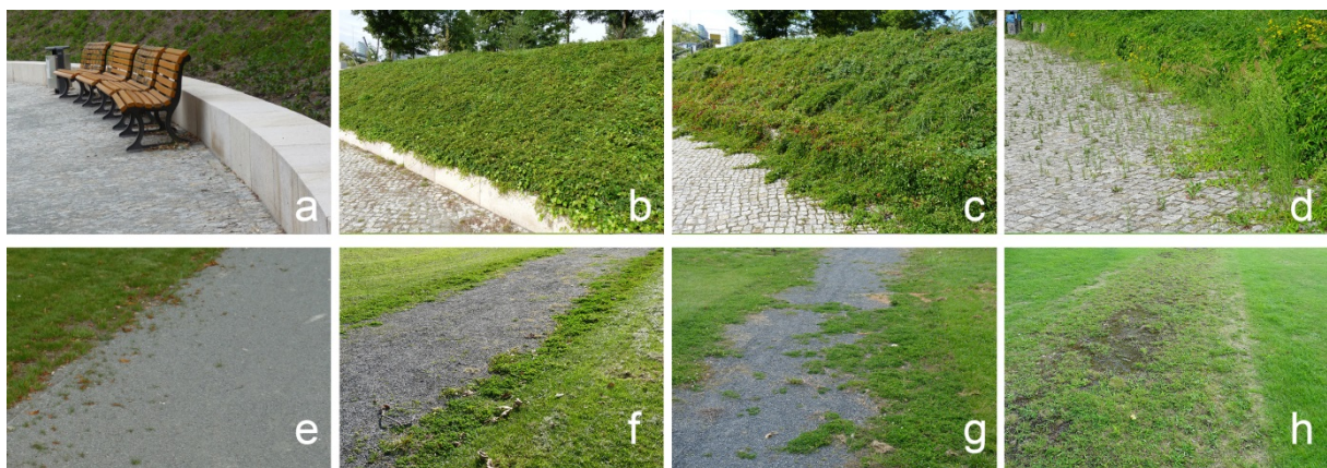
Figure 3: Sequence a-d: The encroachment of planting from embankment onto paving surface over 8 years. a) Year 1. b) Year 2. c) Year 6. d) Encroachment of vegetation promotes further spontaneous growth, Year 8.
