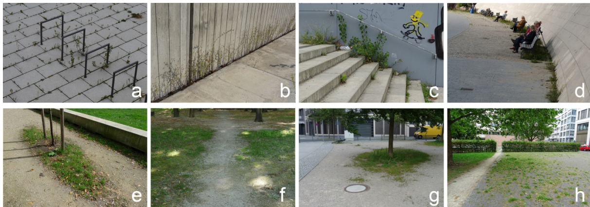
Figure 8: Spontaneous urban growth. a) Growth in jointing material of paving, year 3. b) Vegetation in open joint between surface and wall, year 7. c) Growth in joints of steps, year 7. d) Spontaneous growth in gravel joint at the foot of an inclined wall, year 6. e) Growth surrounding tree in self-binding gravel surface, year 3. f) Self-binding gravel surface in full shade of trees, year 5. g) Tree in self-binding gravel surface, year 7. h) Increased growth in gravel joints of paving beneath a tree, year 8.
