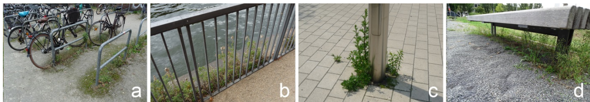
Figure 4: Conflicts around fixtures. a) Impeded maintenance access when in use, year 7. b) Inaccessible spontaneous growth, year 8. c) Growth around street lamp, year 4. d) Hindered maintenance of covered surface, year 7.
