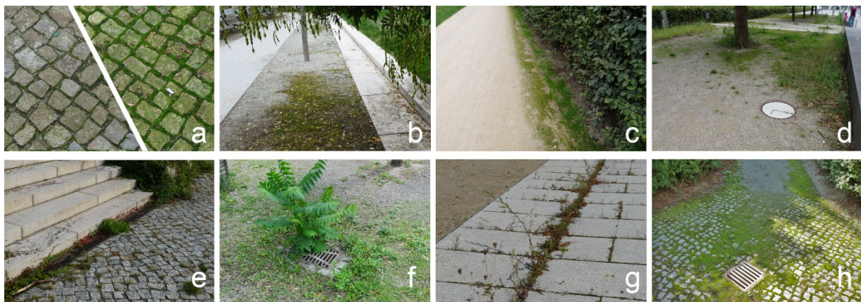
Figure 6: Images a-d: Increased vulnerability to spontaneous growth in shade. a) Limestone setts in full sun/full shade of a building, year 3. b) Increased spontaneous growth due to overhanging tree, year 3. c) Spontaneous vegetation adjacent to hedge, year 3. d) Spontaneous growth on compacted gravel surface below tree, year 4. Images e-f: Conflicts with drainage elements. e) Encroachment of vegetation from neighbouring embankment, year 3. f) Growth within gully in compacted gravel surface, year 8. g) Blockage of slit drain due to organic debris and spontaneous growth, year 3. h) Minimal gradient leading to sedimentation and growth on surface, year 10.
